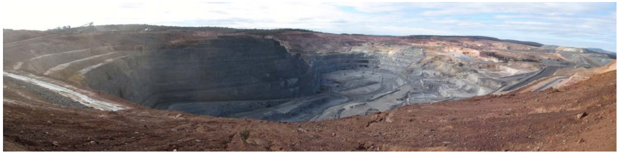
The South pit at Newmont's Boddington operation May, 2011 (Photo by Alfonso Rodriguez)
