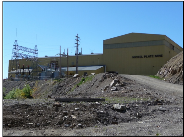
The former mill and current water treatment plant.
