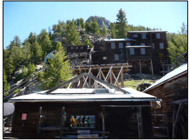
Looking from the blacksmith shop (foreground), to the cookhouse, the smaller miner's dry, and the white tramline wheelhouse.
